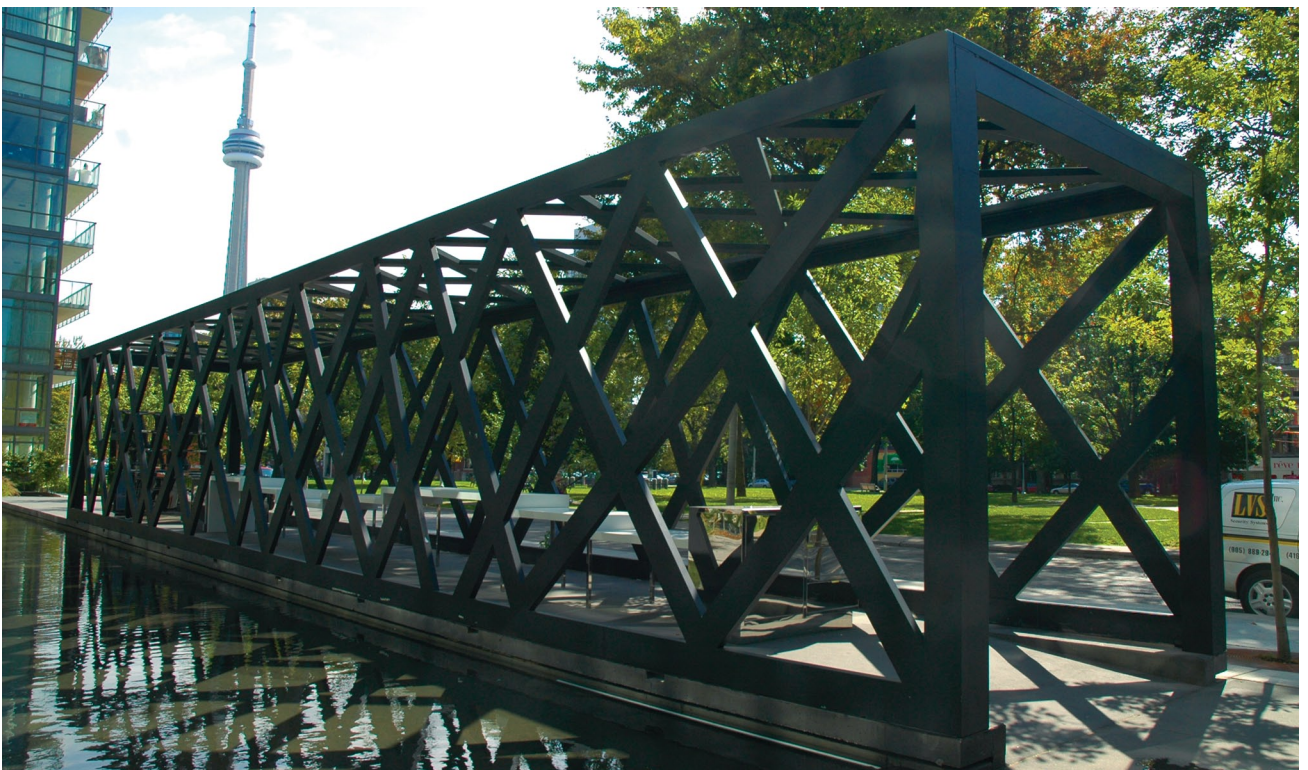
The trellis pavilion at 550 Wellington Ave
