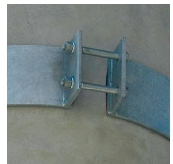
Solid, bolted lap joint connection
