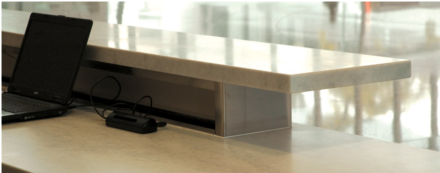
Detail of the marble and stainless steel, raised transaction counter
