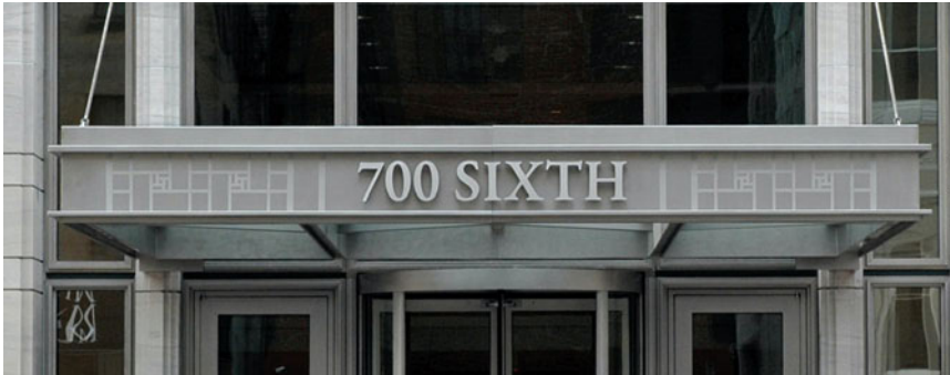
Exterior stainless steel canopy cladding
