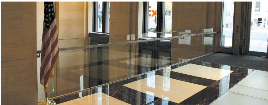
Glass balustrade and railings over the concourse
