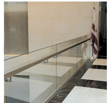
Balustrade and handrail detail
