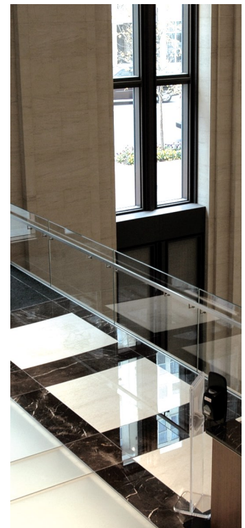
Glass floor and balustrade from above
