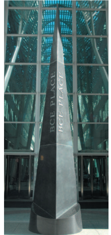
St. stl. letters pinned mounted on granite obelisk
