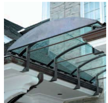
Designed to integrate with existing structure
