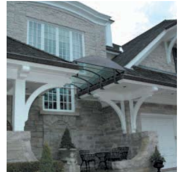
Designed, engineered and installed by SML
