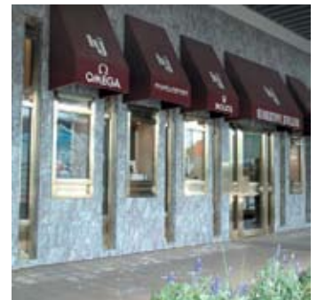
(4) windows and entrance door
