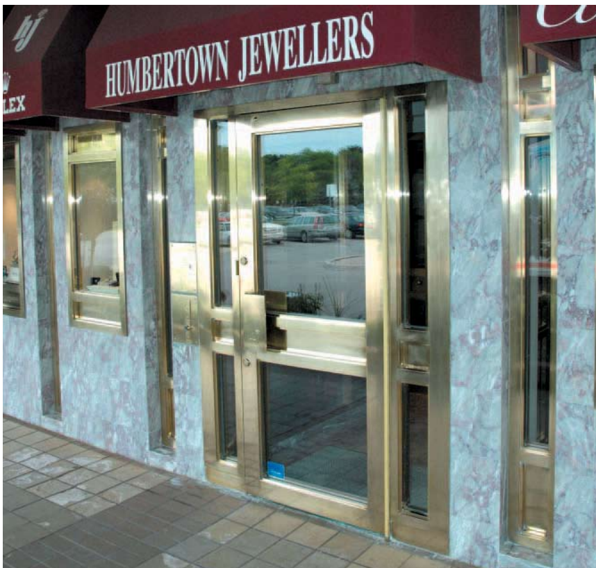
Bulletproof glass and solid structure ensures security
