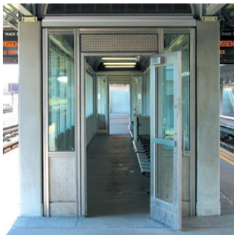
Cabins - approx. 9' wide by 60' long
