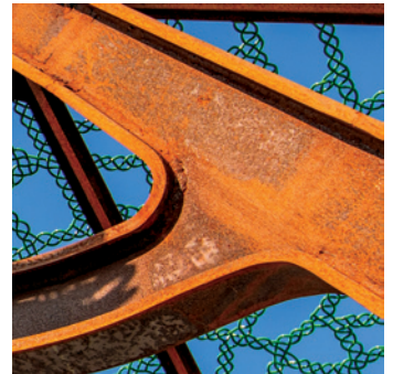
Detail of the COR-TEN steel forming work
