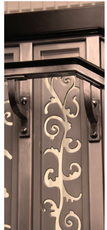
Detail of panel, railing and fasteners.
