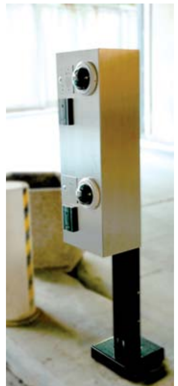
Security camera post & card access enclosure
