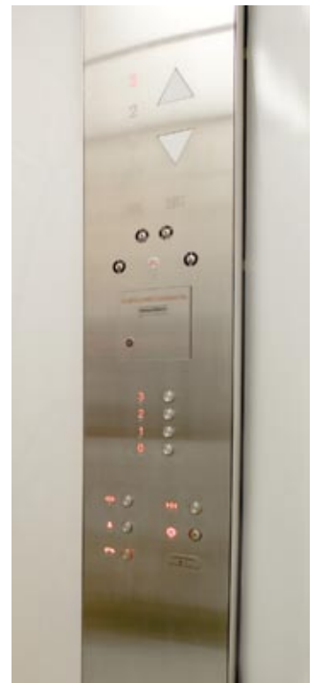
Stainless steel control operating panel (COP)
