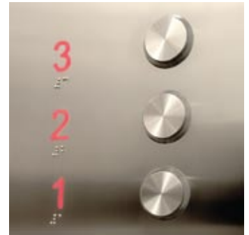
Detail of the COP with braille embossing
