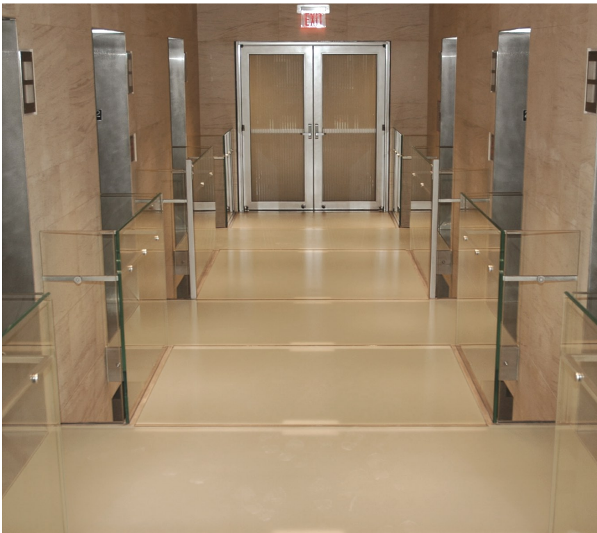
Glass bridge services elevator entrances
