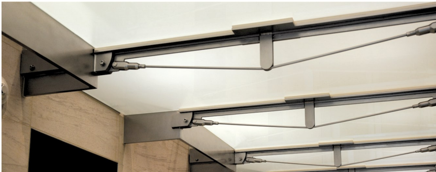
Stainless steel rods and adjustable clevis support system
