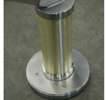
Brass and steel footings
