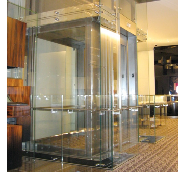
Stainless steel and glass elevator shaft
