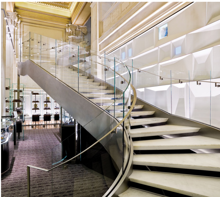
The monumental grand staircase featuring marble treads, stainless steel structure and railings with glass balustrade
