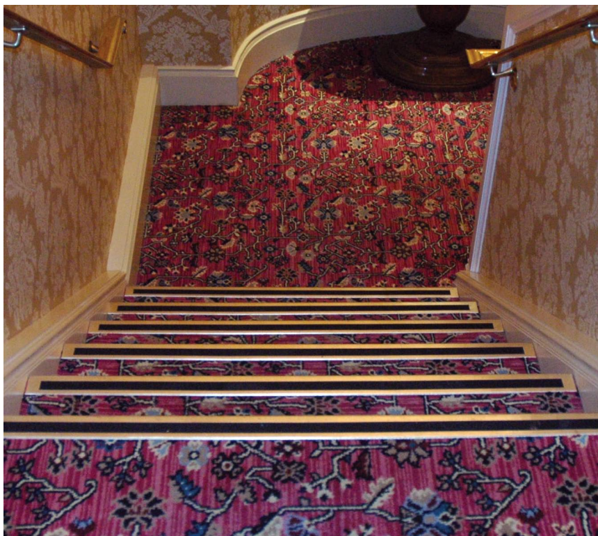
These custom made bronze stair nosings add safety and elegance to a well used staircase
