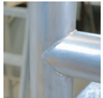
Strong structural weld
