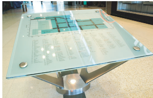
1" thick stainless steel support legs
