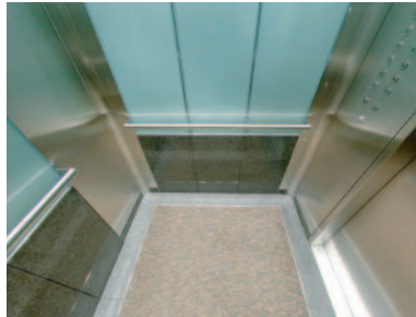
Granite walls and floor panels with inlay carpeting
