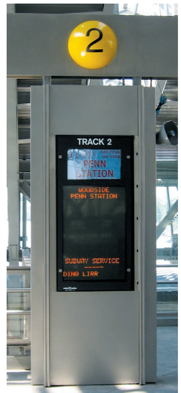
Stainless steel cladding and LED signboard
