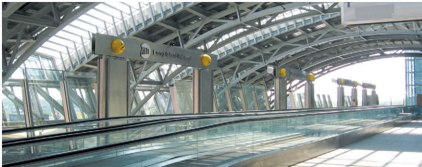
Array of girders spanning approximately 150 feet
