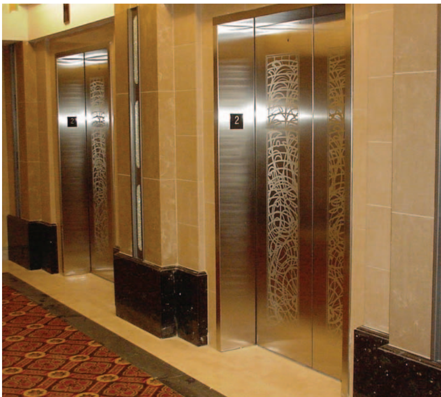
Etched elevator door panels
