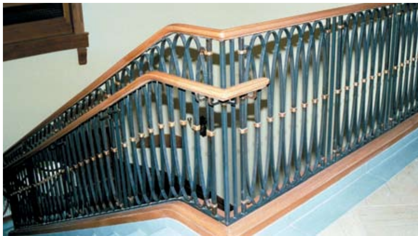
Guardrail and handrail
