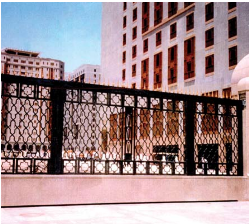
Close up of completed fence section
