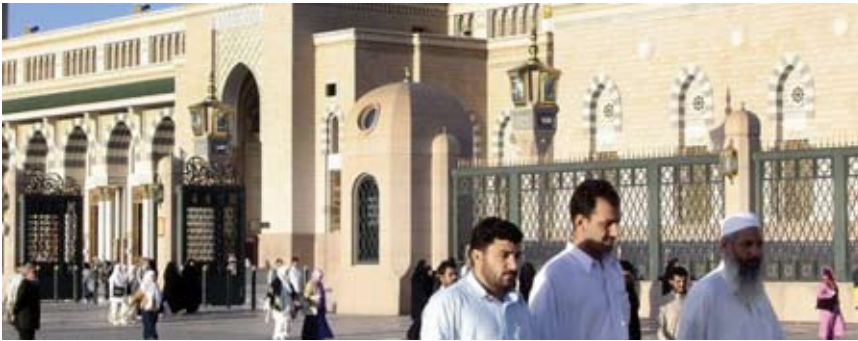
The completed fences and gates at the entrance to The Prophet's Mosque.
