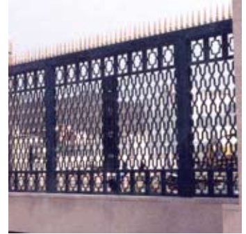
Completed fence section
