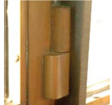
Alloy 230 custom made red brass hinges
