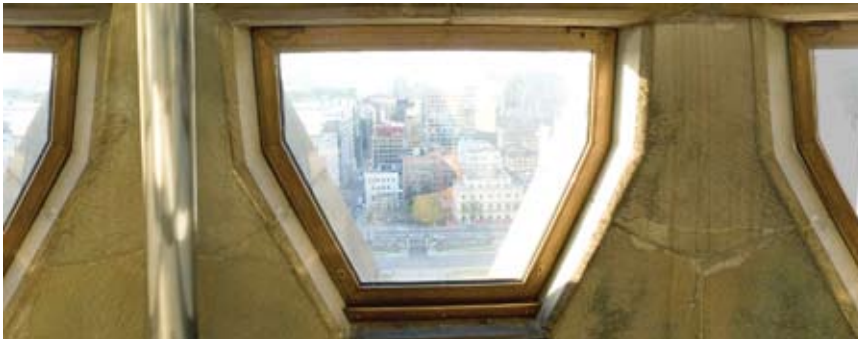
Custom crafted trapezoidal bronze windows surround the lower portion of the observation deck
