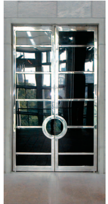
A set of st. stl. entrance doors, interior
