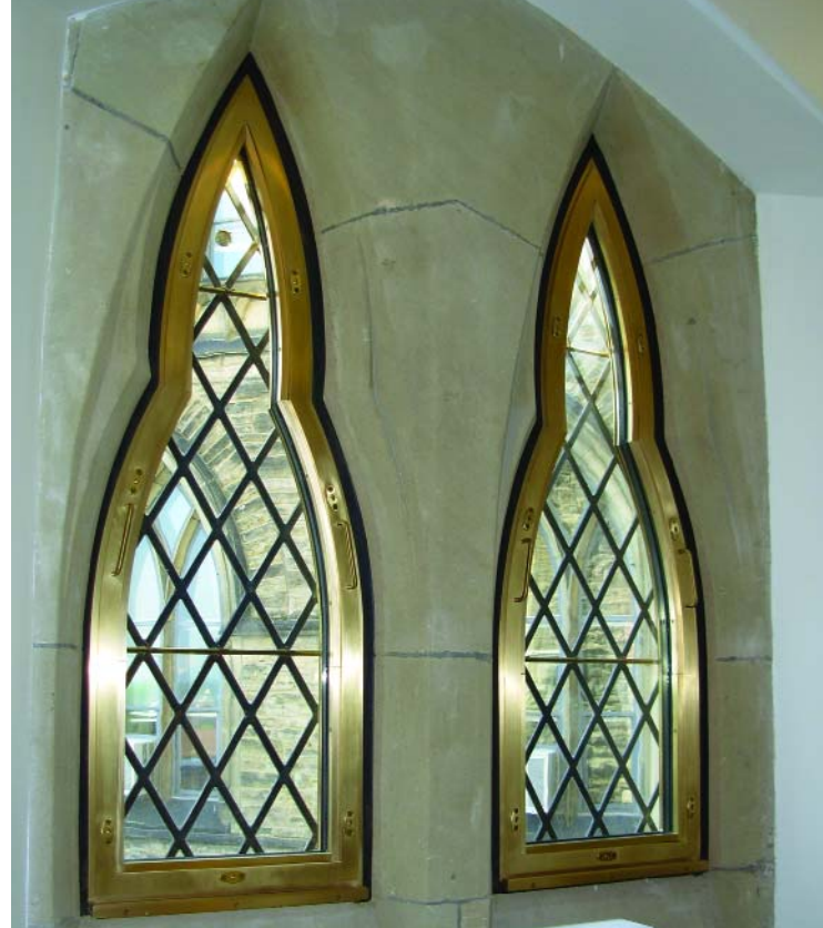
▲ 207 bronze windows were produced and custom tailored for each opening.
