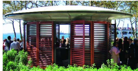
▲ The kiosks were oval shaped; made from Jatoba wood, glass, and stainless steel; and were 20 feet long.
